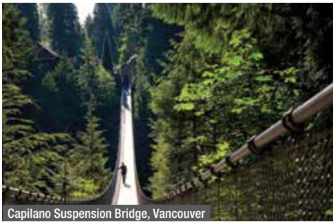
Capilano Suspension Bridge, Vancouver
