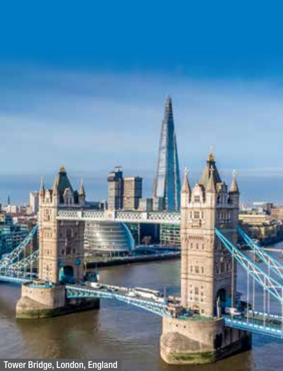
Tower Bridge, London, England
